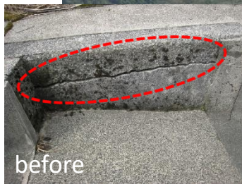
集水桝ひび割れ補修
