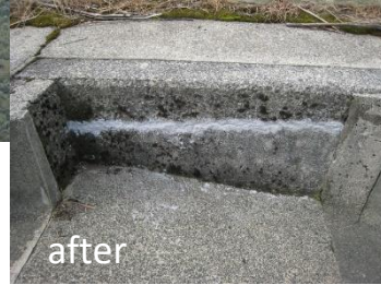
集水桝ひび割れ補修
