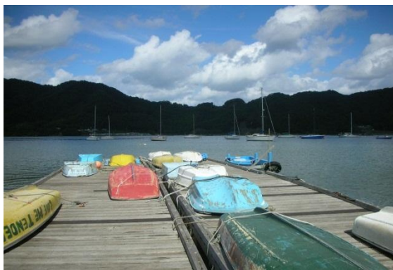
[甲ヶ崎泊地の浮棧橋]
