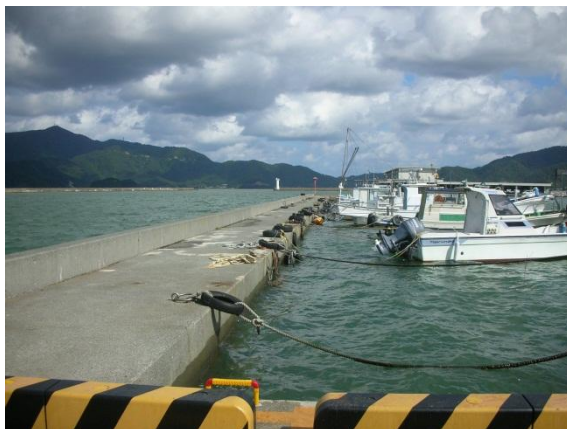
[川崎護岸の係留施設]
